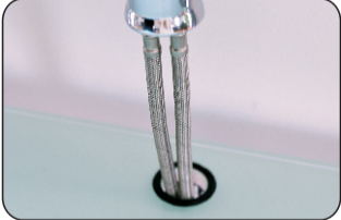
Pass two waterlines through faucet hole of countertop & adjust faucet
