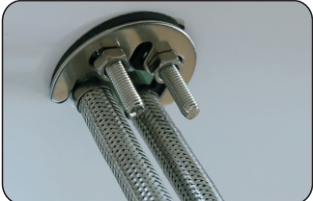
Put nuts on & tighten nuts
