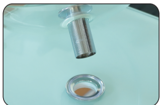
Align the sink with the drain hole and set it up
